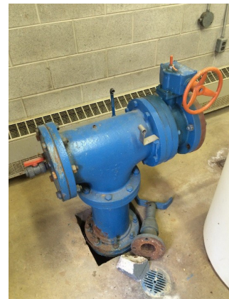
Figure 2. Connection point into existing G11 piping
